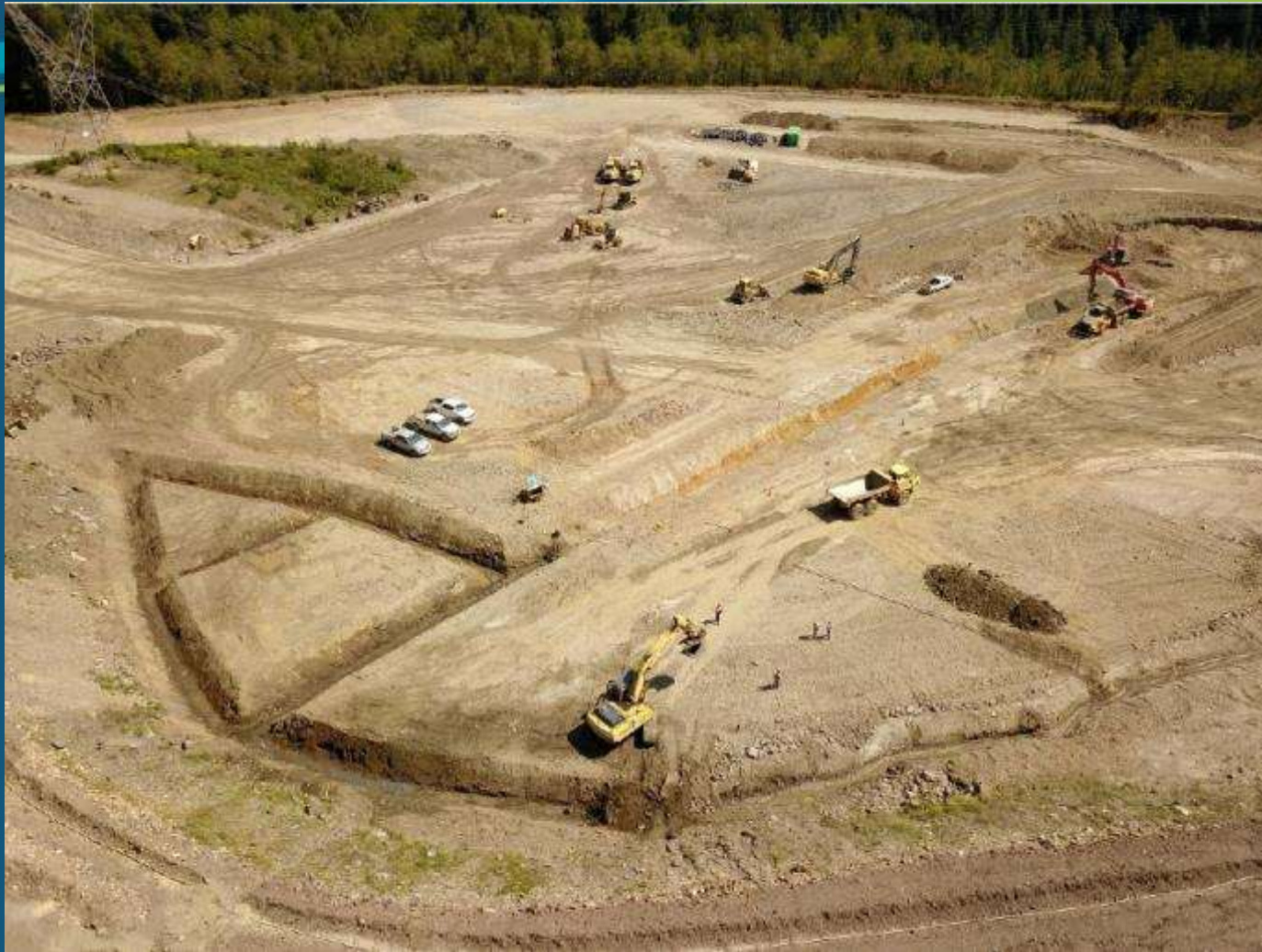
Finger drain construction
