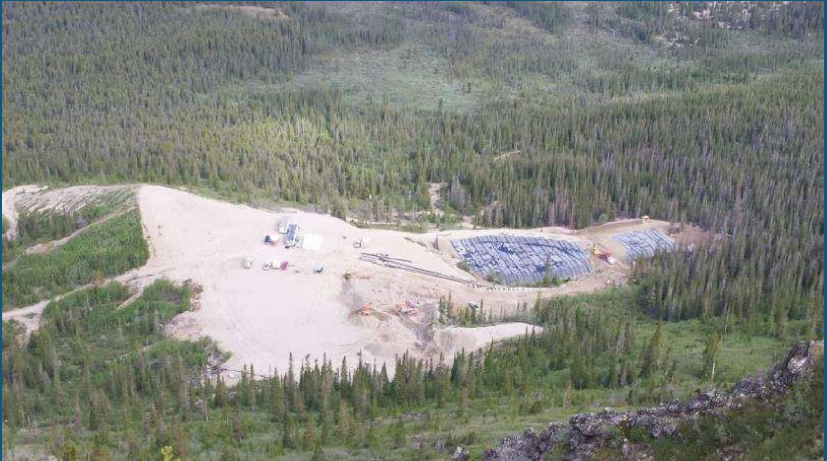
Site during remediation works - 2017
