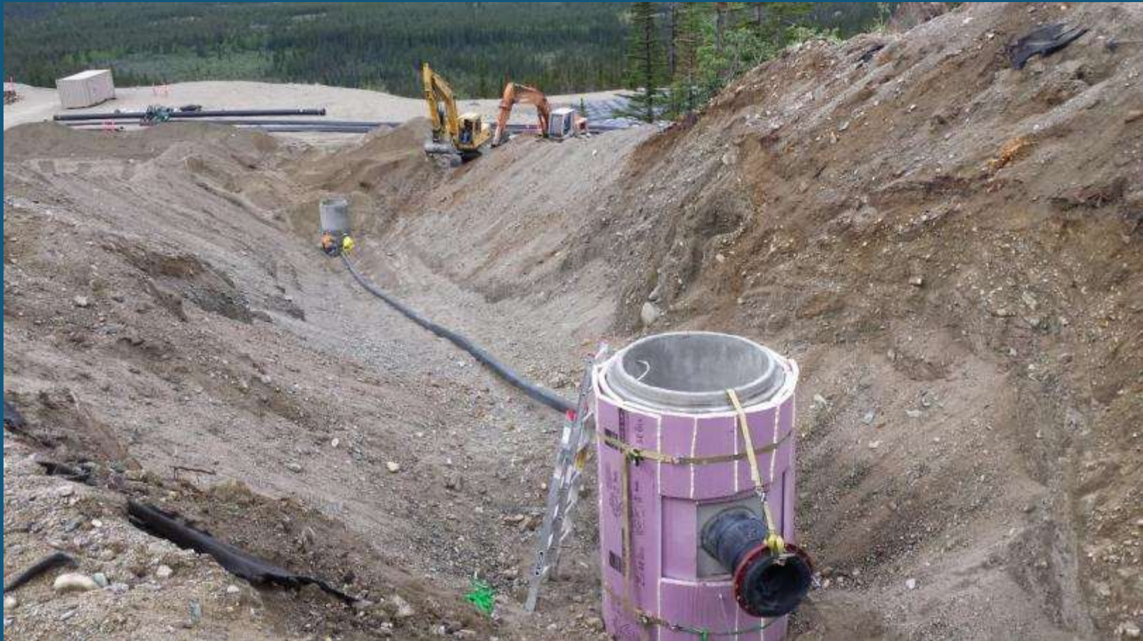
Installation of piped surface water diversion
