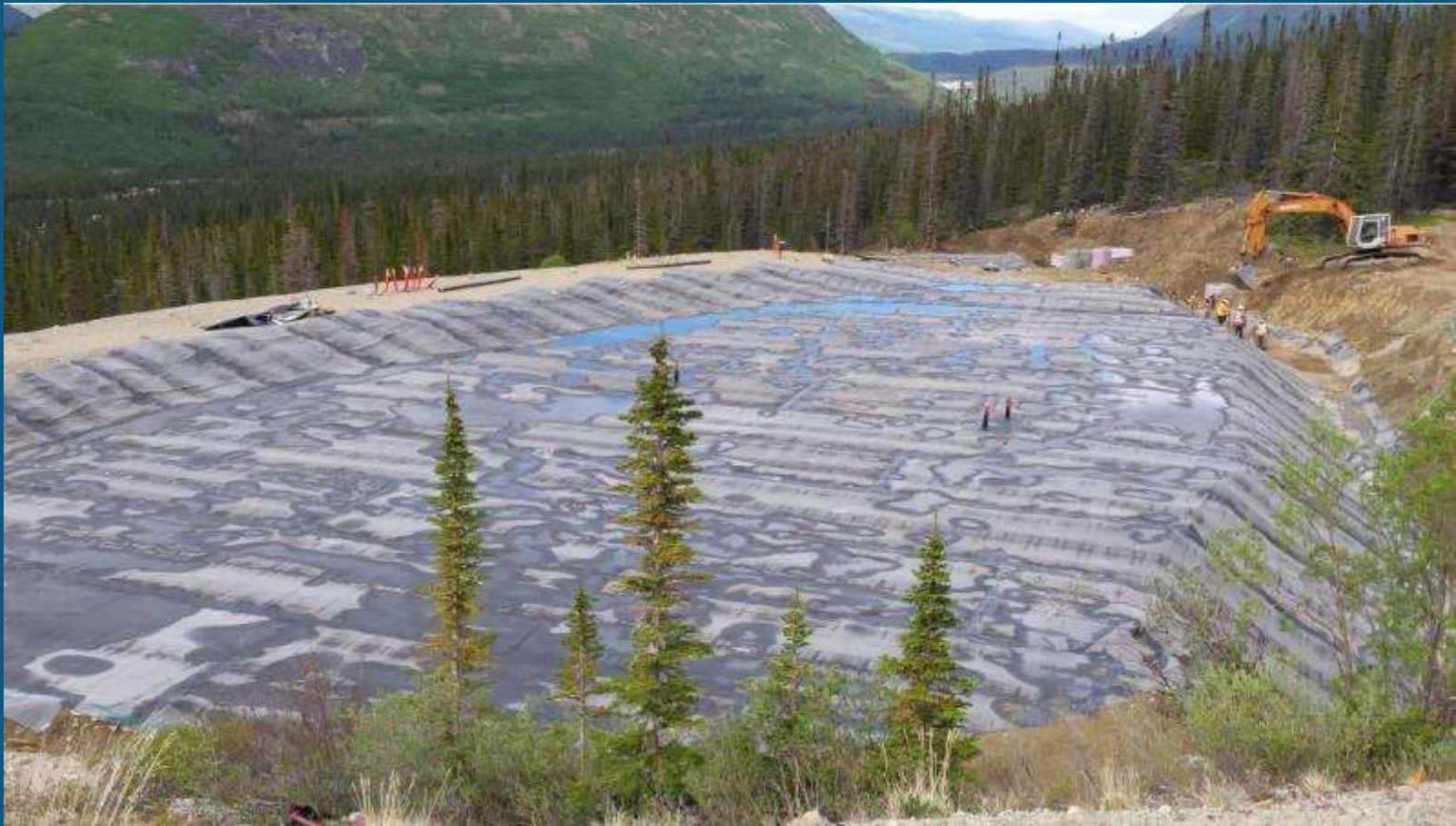
Bituminous geomembrane liner and interceptor trench installation - 2017
