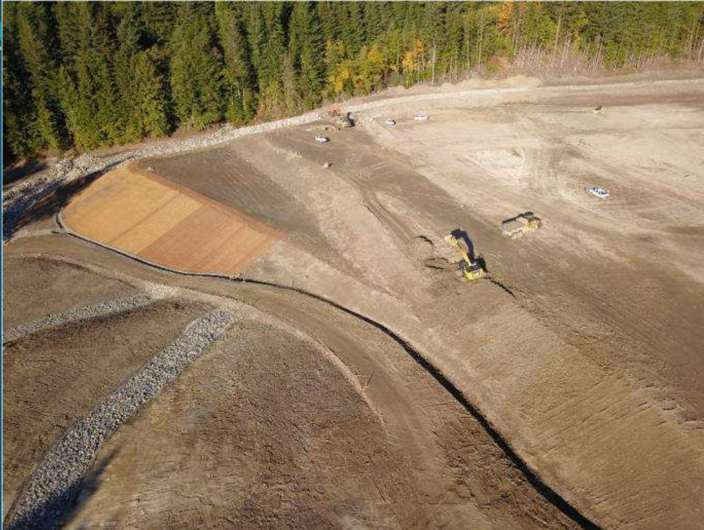
Upper TSF South Embankment
