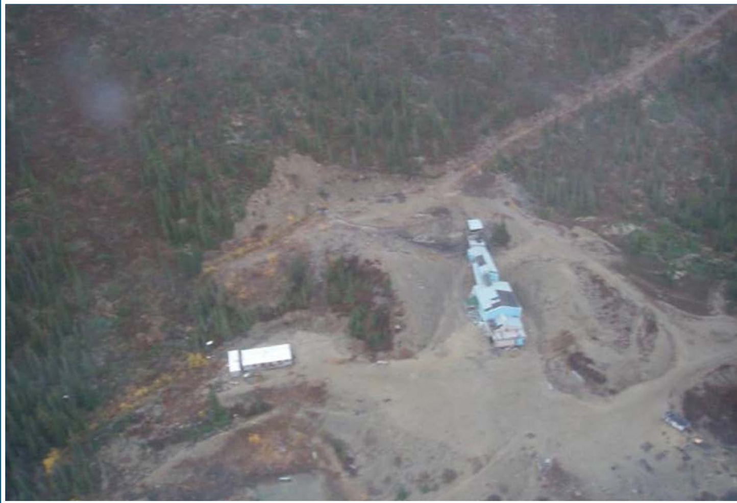
Mill building, trailers and mill pads prior to reclamation (2008).
