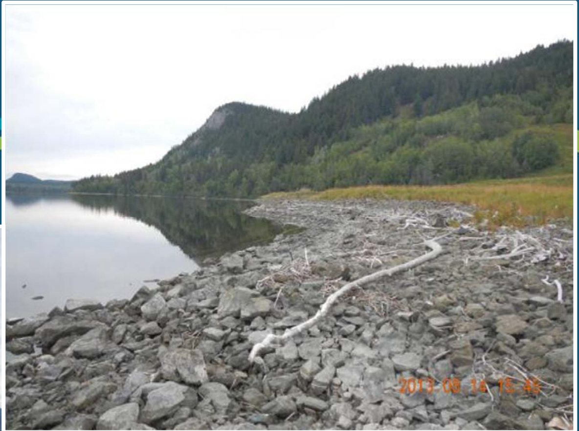
Rip rap protecting calcine waste (2013).
