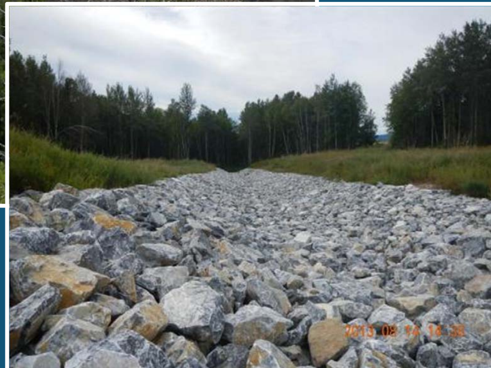
Active tailings impoundment spillway.
