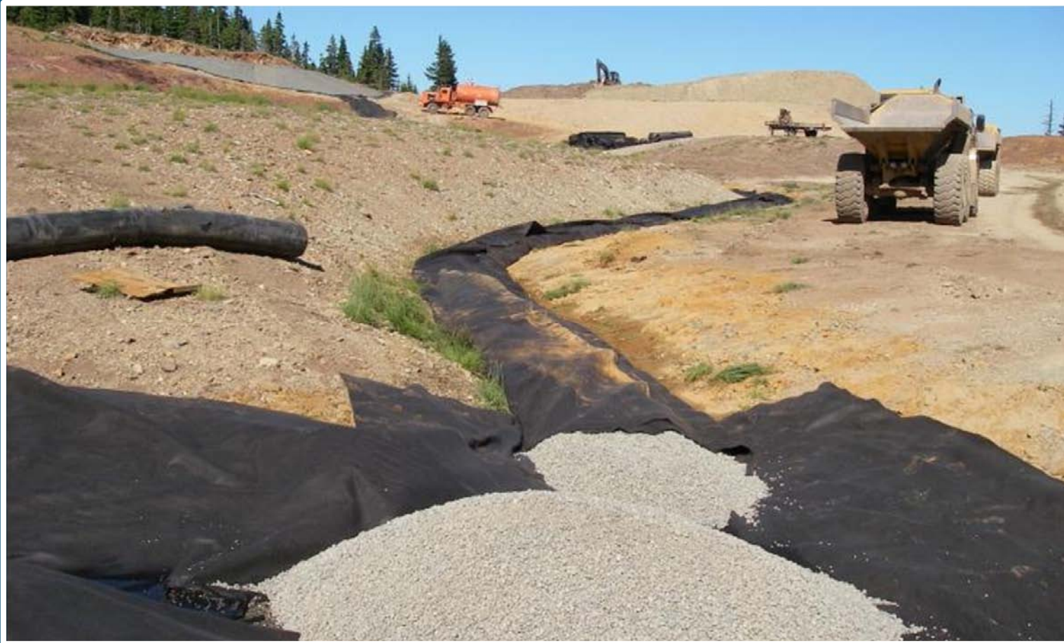
Underdrain Construction
