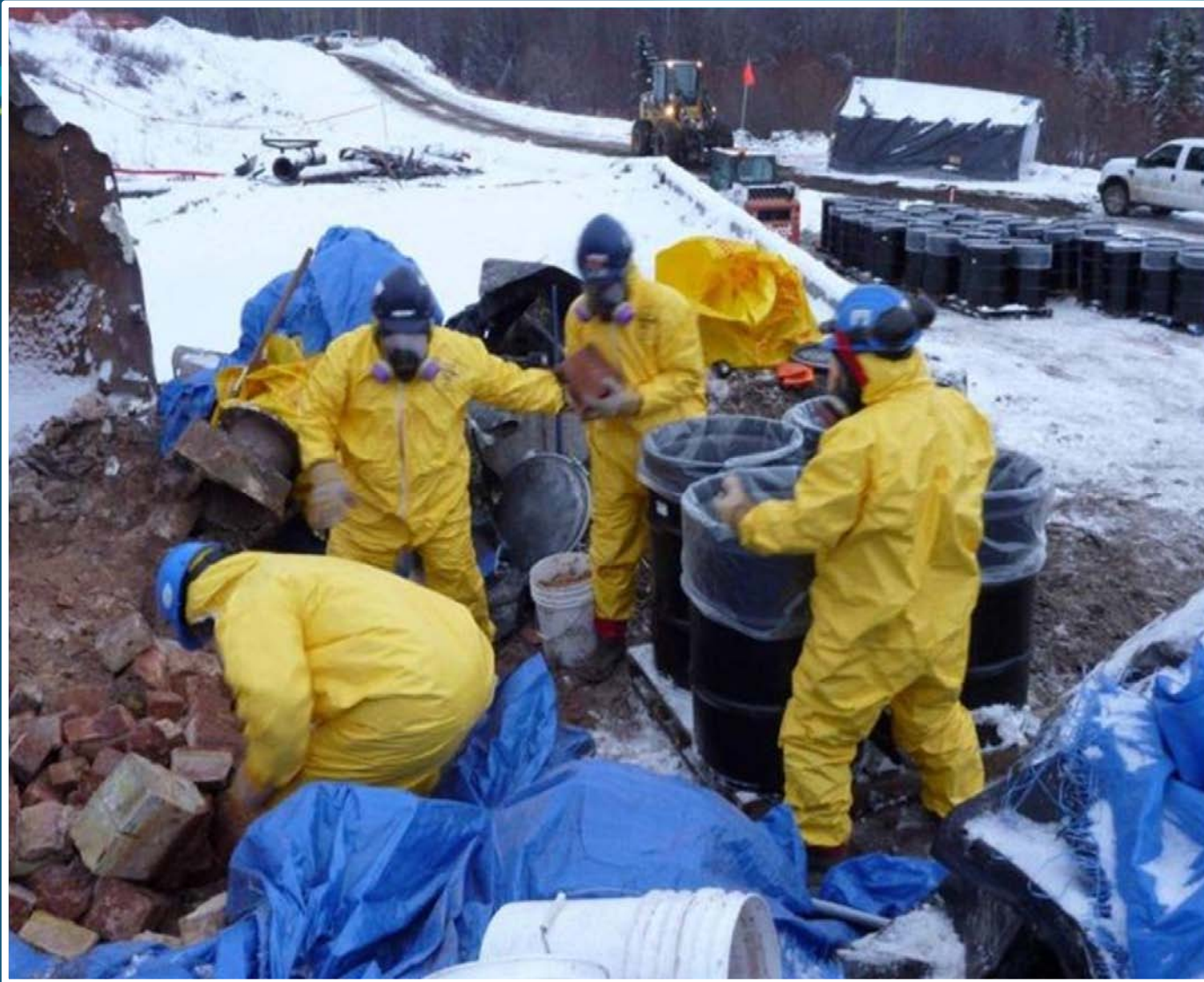
Workers preparing roaster soot and brick work for offsite disposal.
