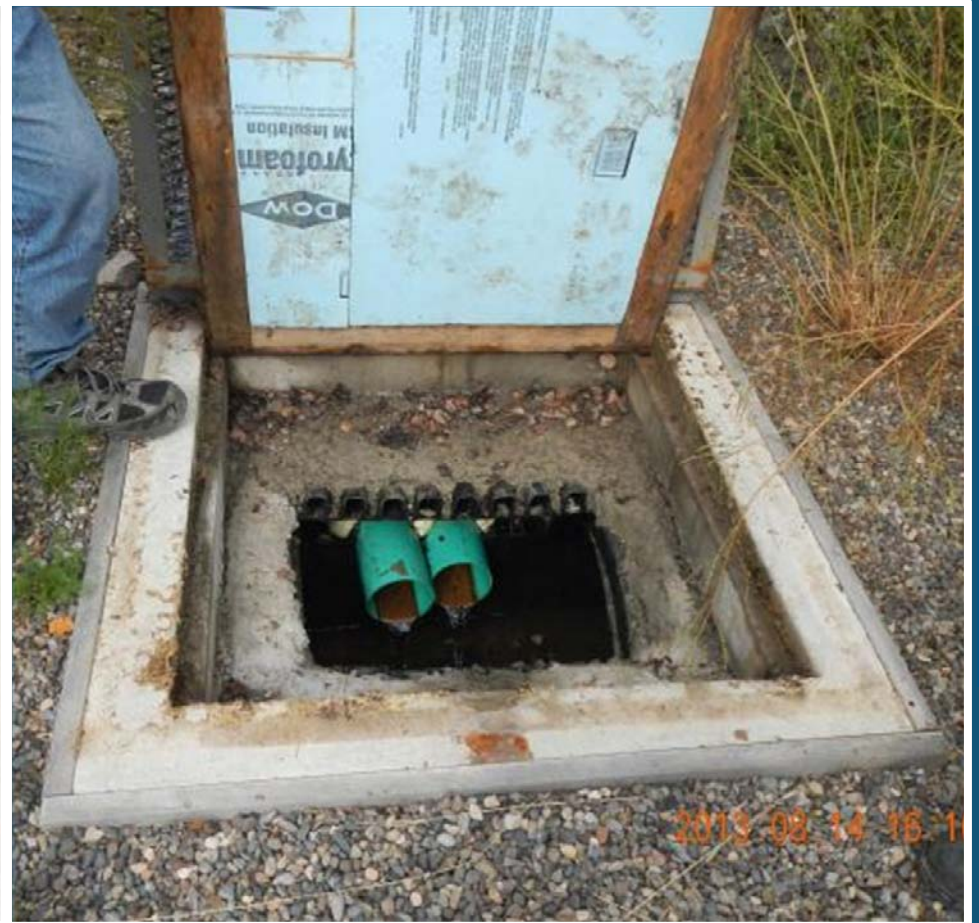
750 portal closure (left) and 750 portal drainage monitoring (right).
