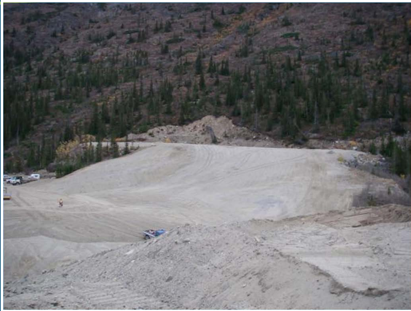
Remediation in progress at the former mill site (September 2012).
