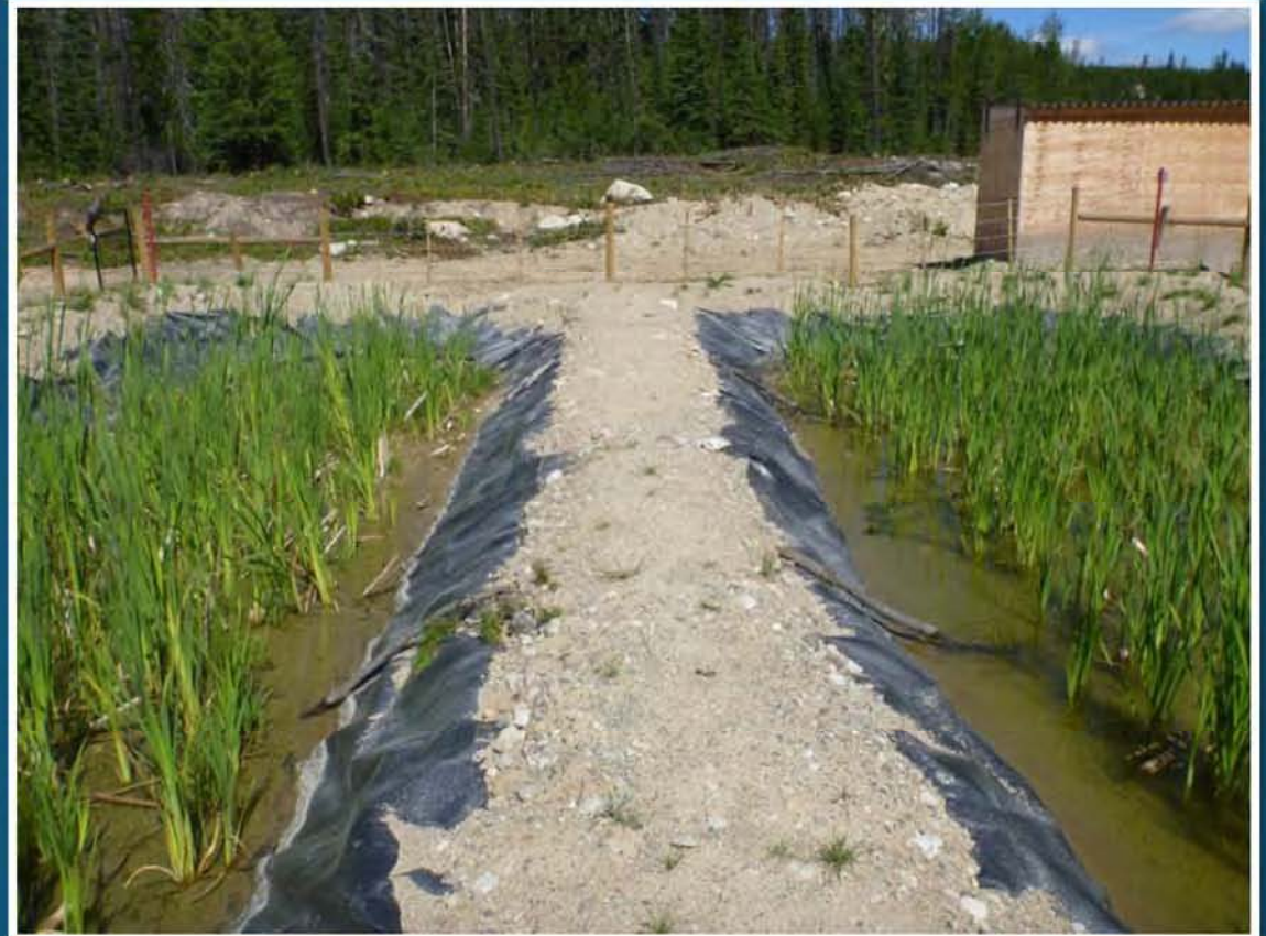
Trial Wetland Construction, Fall 2011 to Summer 2012.
