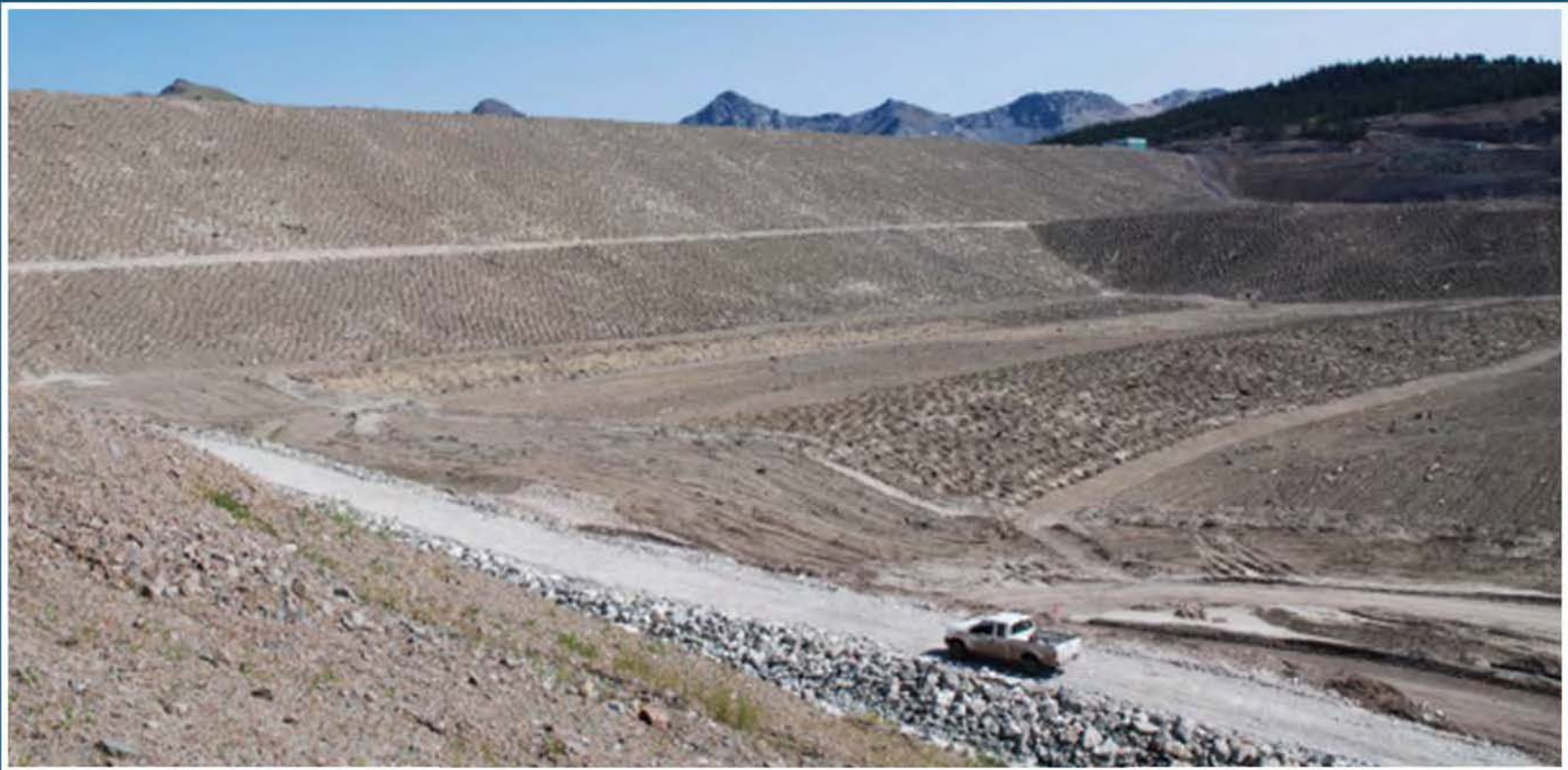
Final dam surface, August 2009
