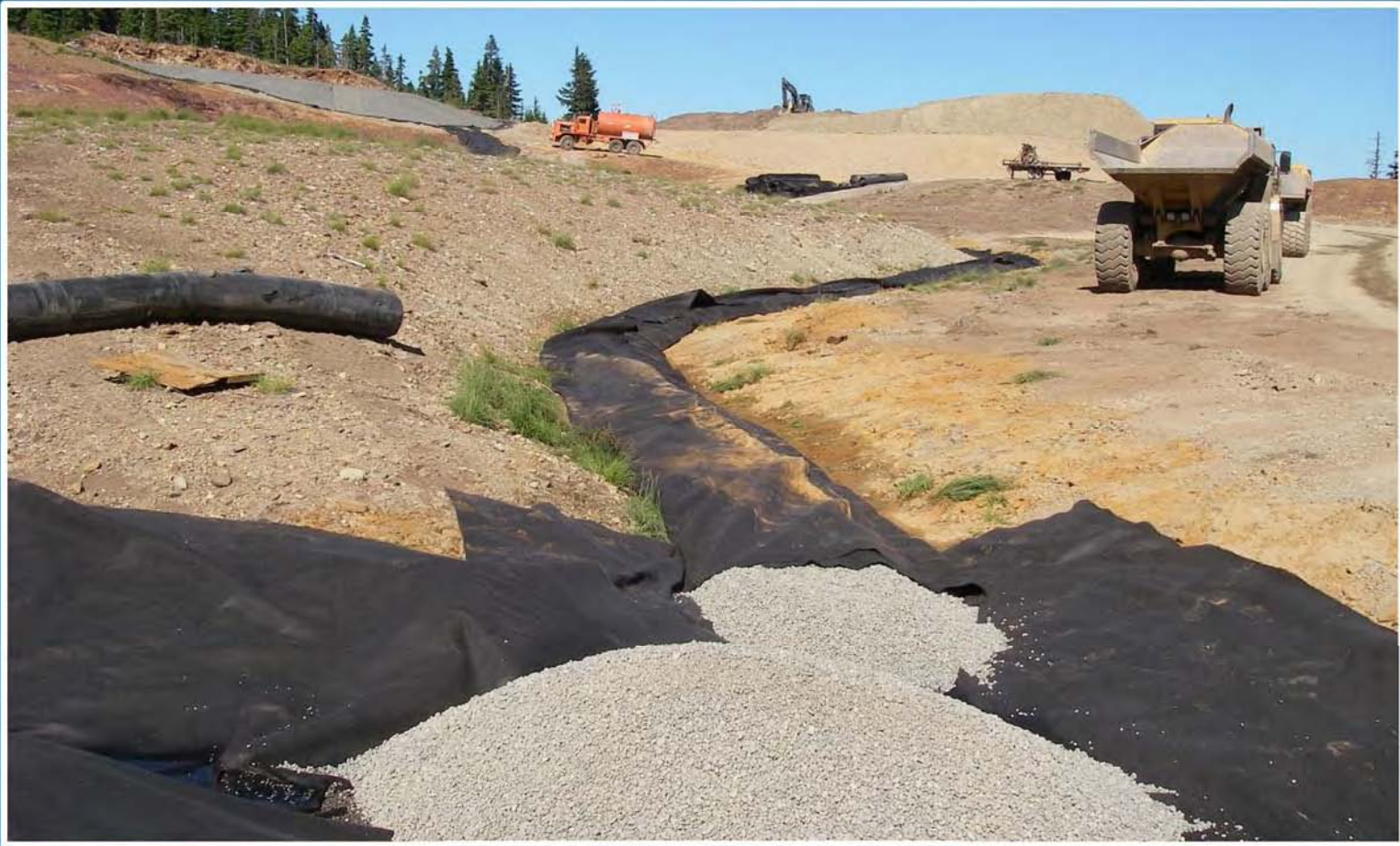
Underdrain Construction
