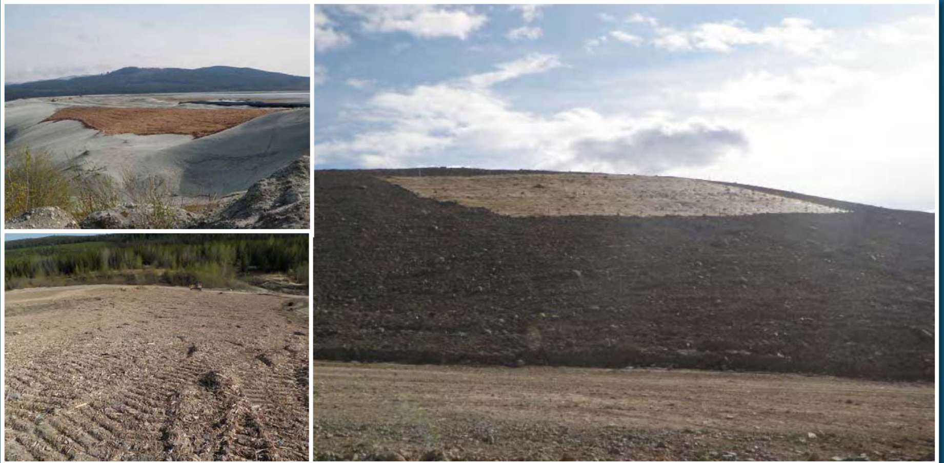
Main Sand Dam, with placement of wood chips (left), and pine tree establishment trial (2011).
