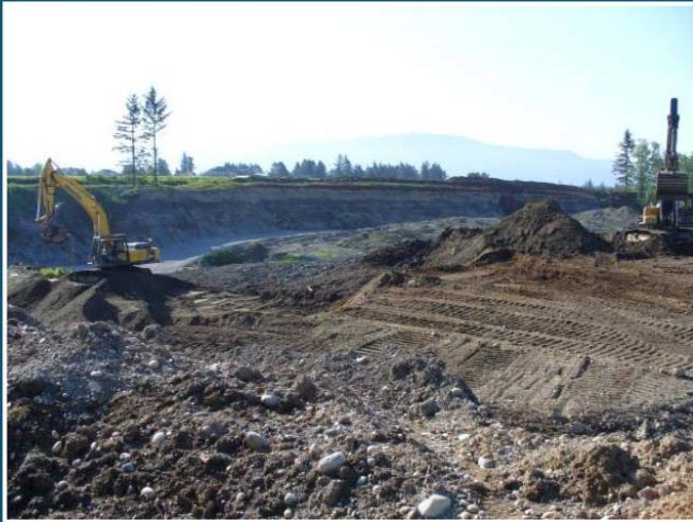
Clean construction fill backfilling (early stages)
