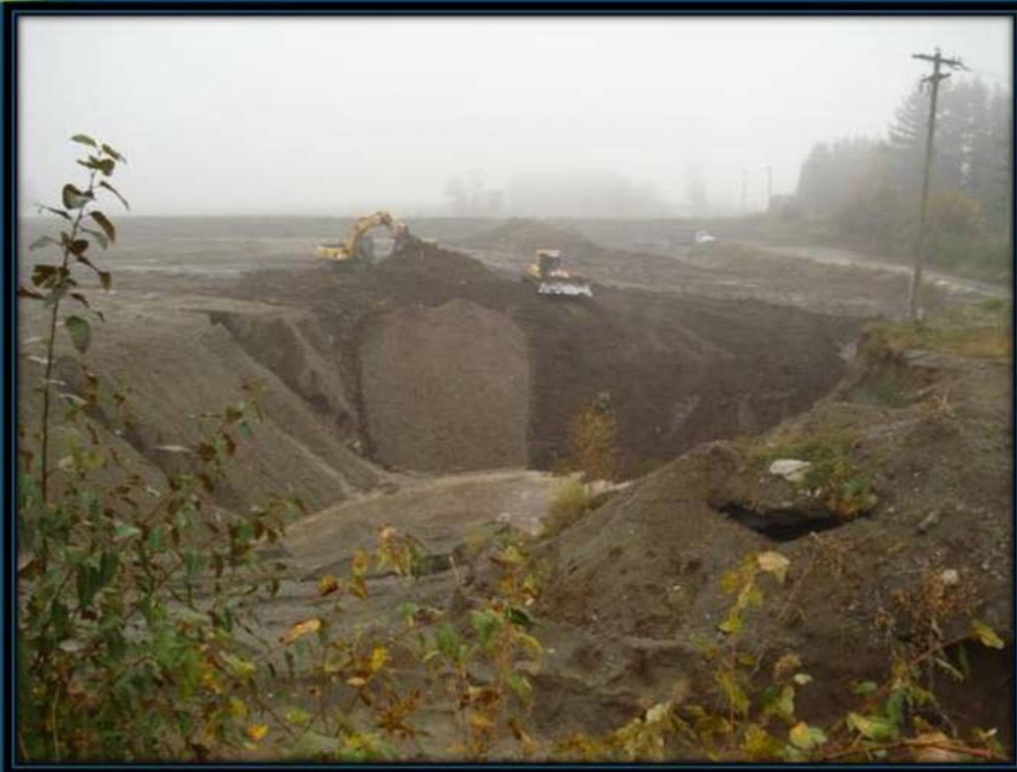
Clean backfilling progress (2009)
