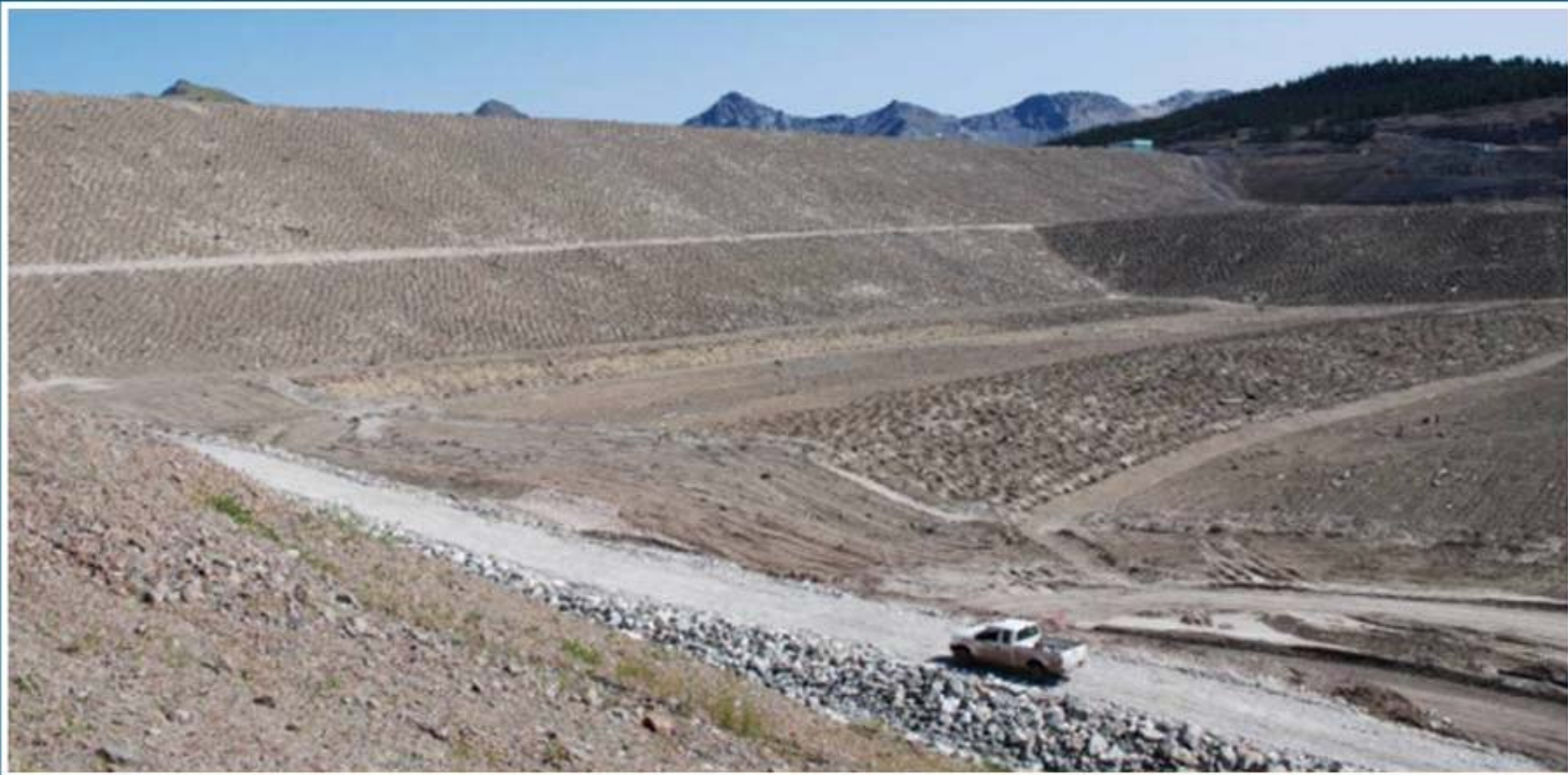
Final dam surface, August 2009
