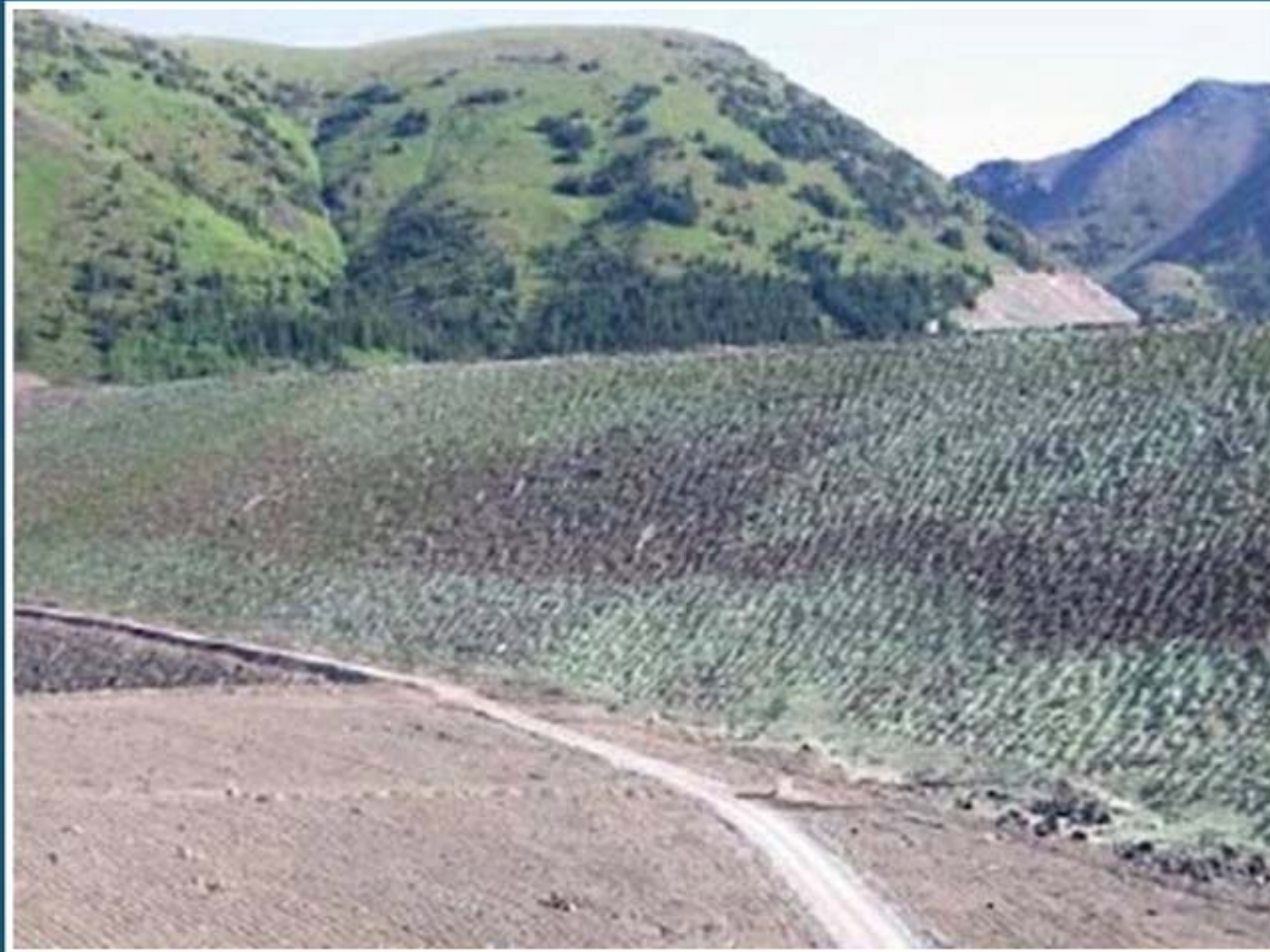
Hydroseeding in progress on dam face (August 2011)
