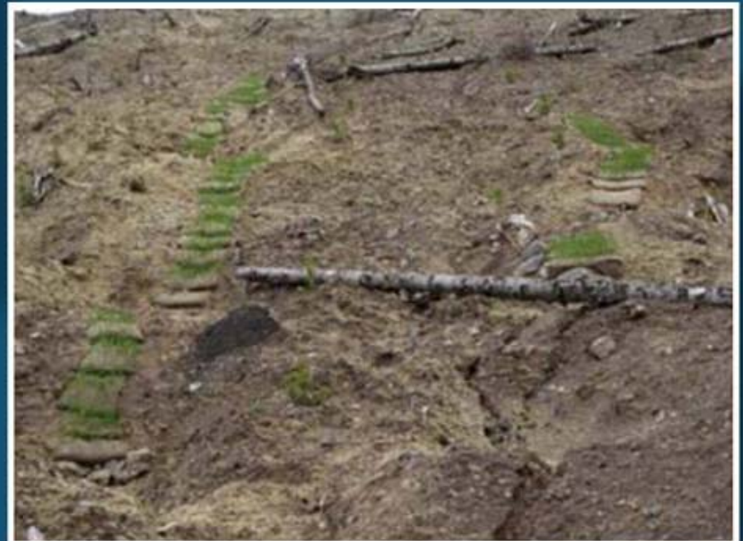
Peat and barley filled burlap armouring on dam face (August 2011)
