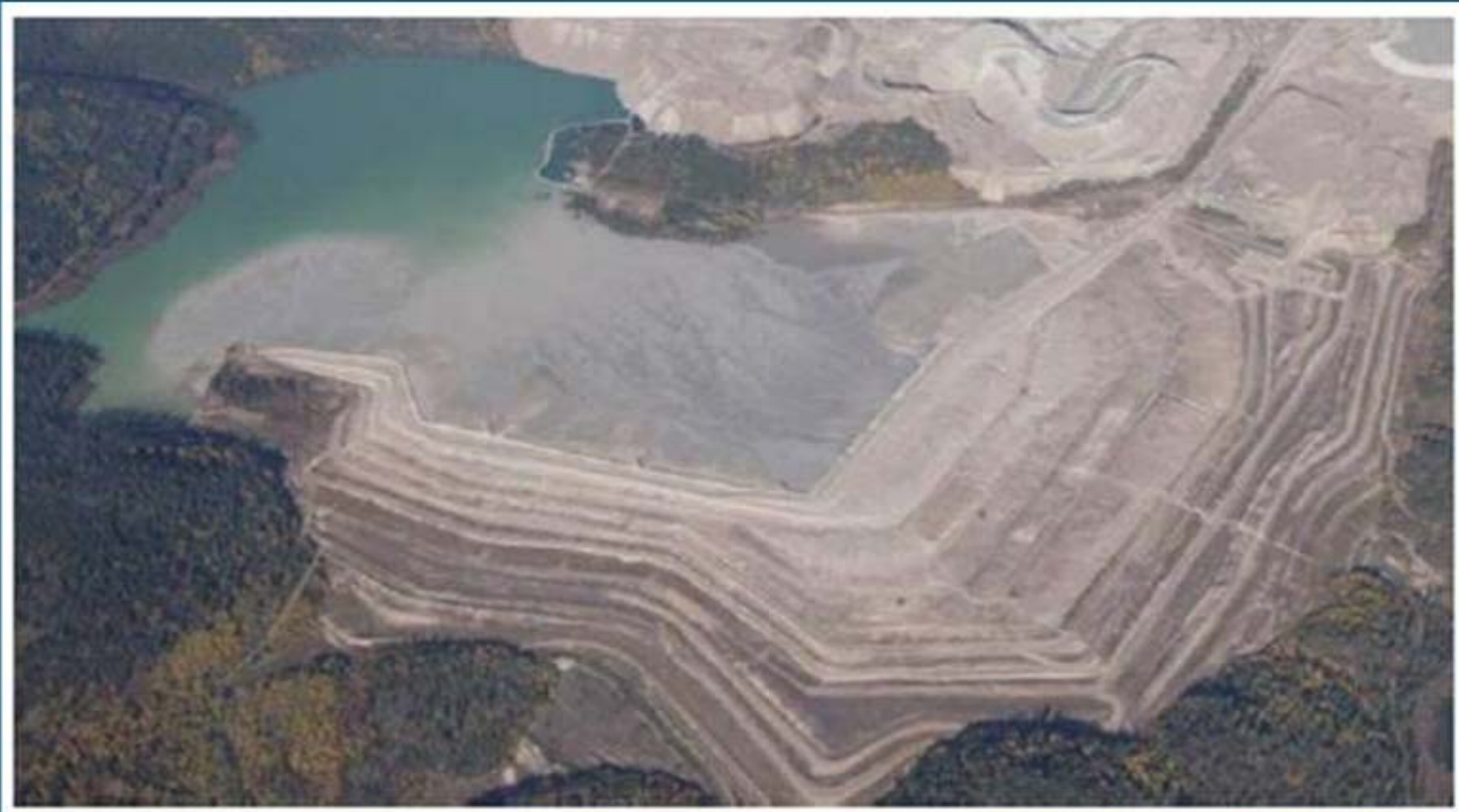
Tailings dam embankments of coarse tailings sand
