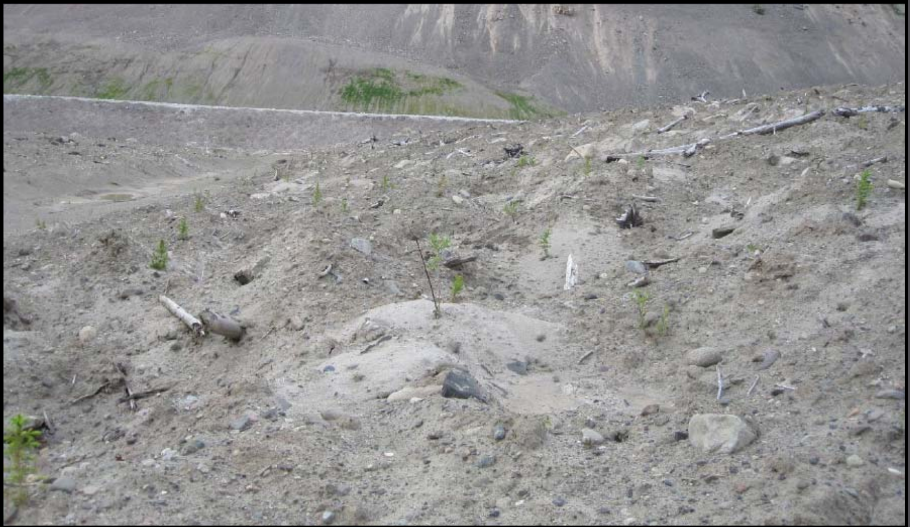
Dam buttress surface, July 2010
