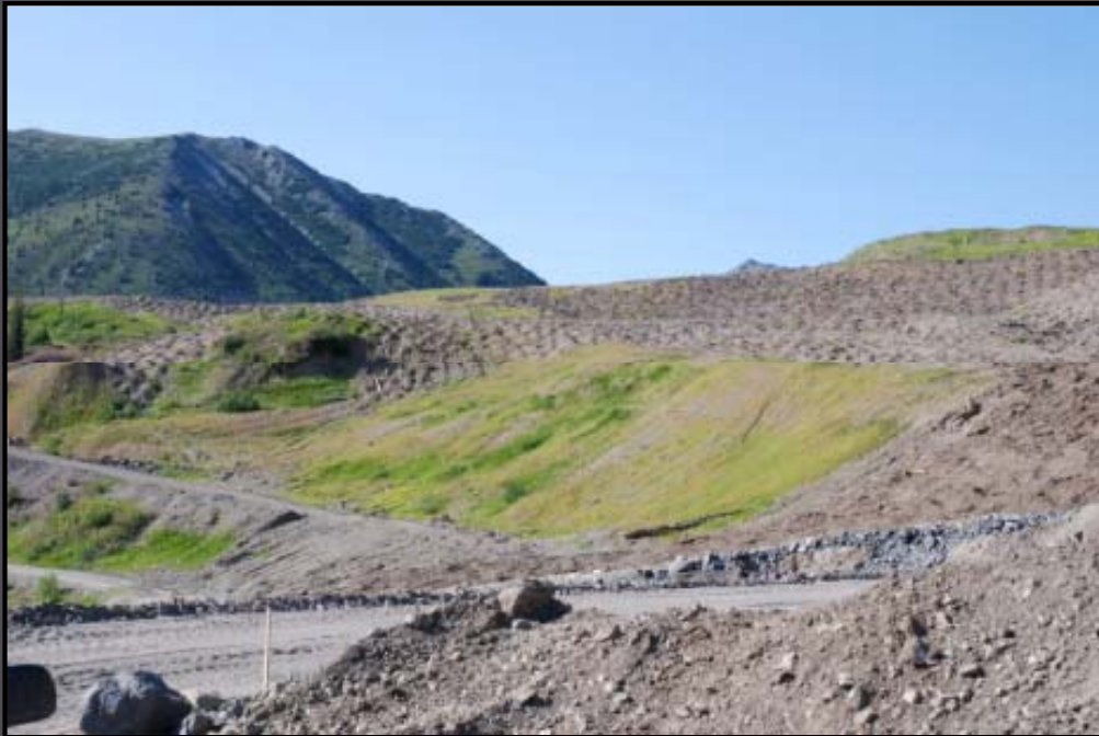
Loose and rough soil preparation
