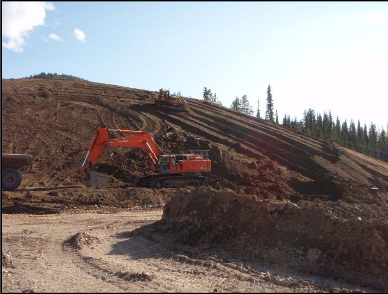
Waste rock surface preparation and overburden placement (July, 2010)
