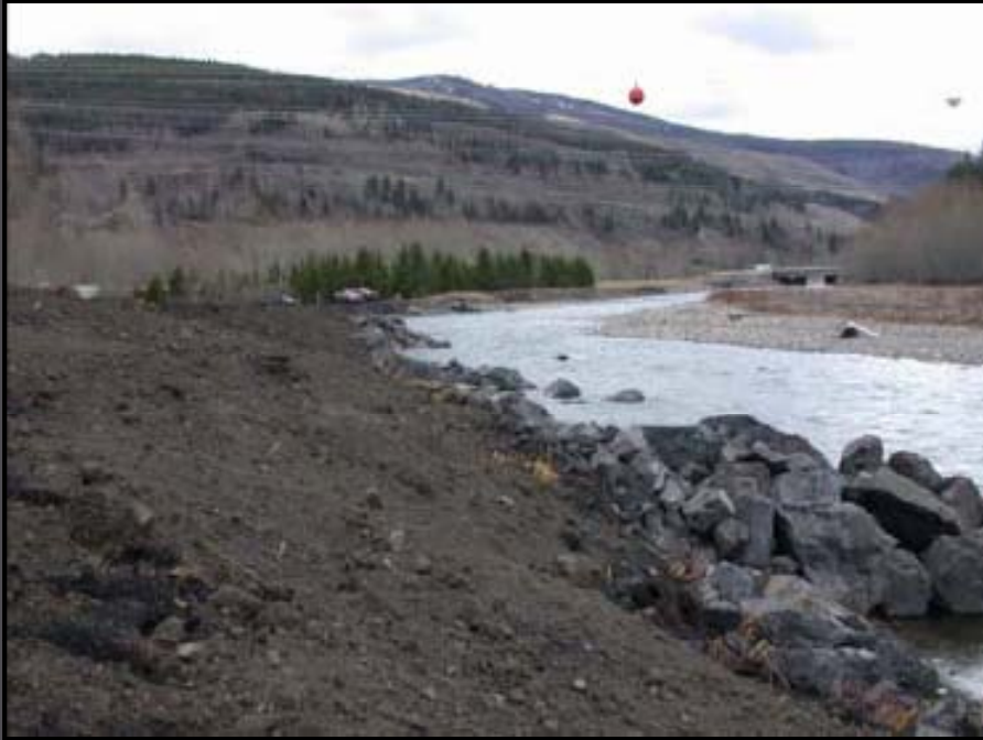
Streambank following construction (April 2004)
