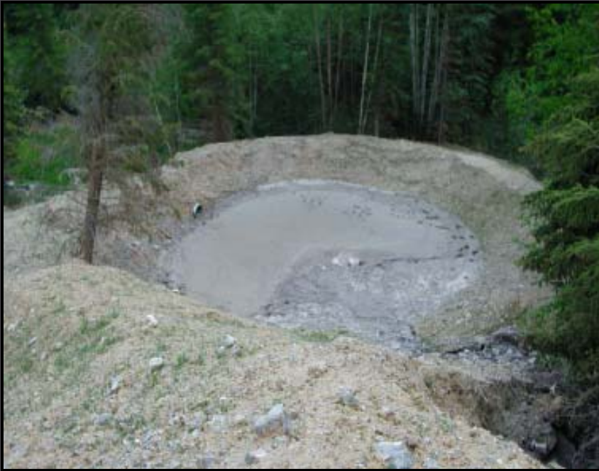
Sediment control pond
