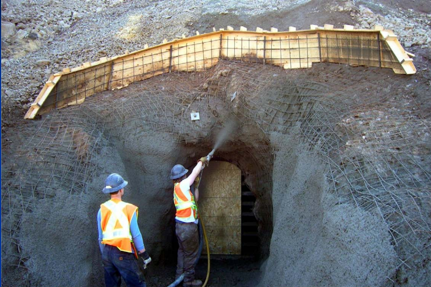
Shotcrete Application at Adit 2
