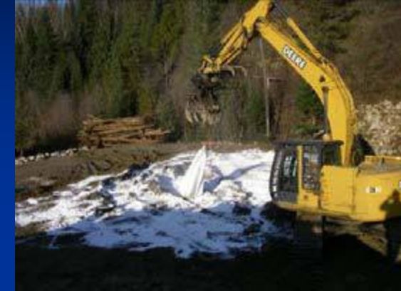
Lime Addition to Neutralize Tailings
