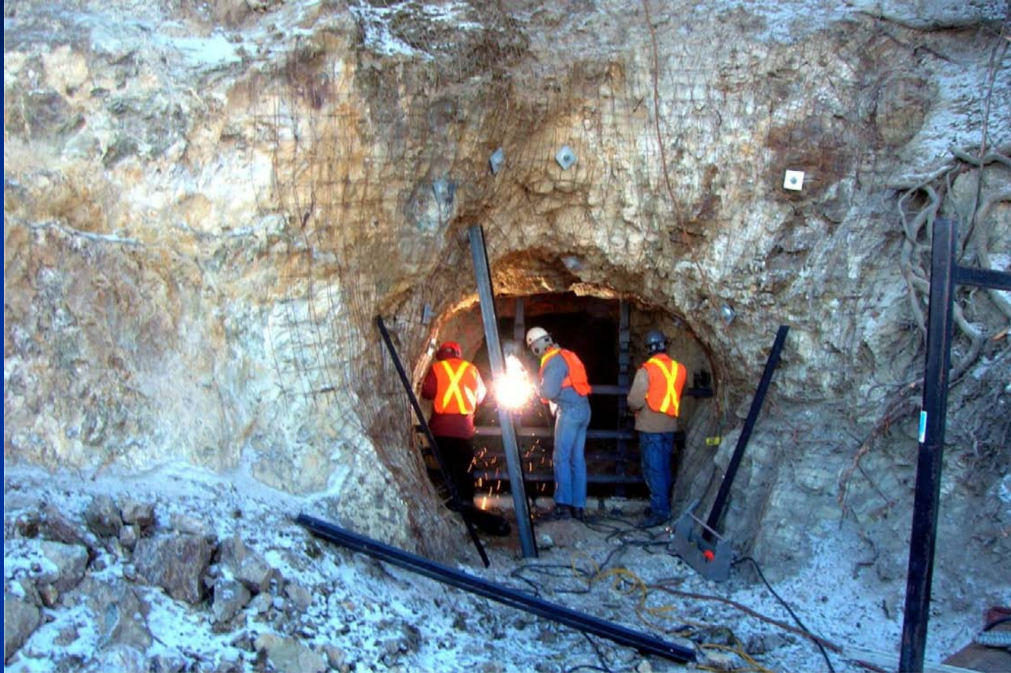
Installation of Bat Gate on Adit 1
