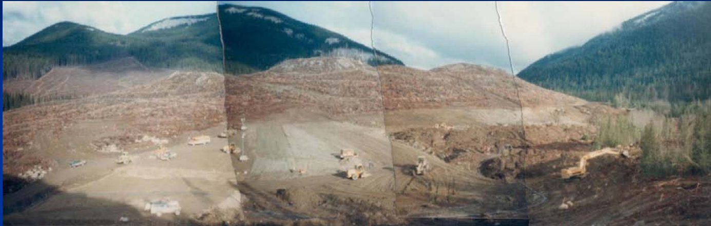
Early mine construction
