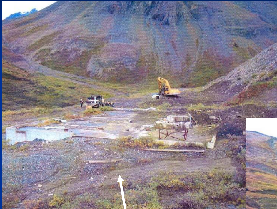
BEFORE Mill Building Foundation
