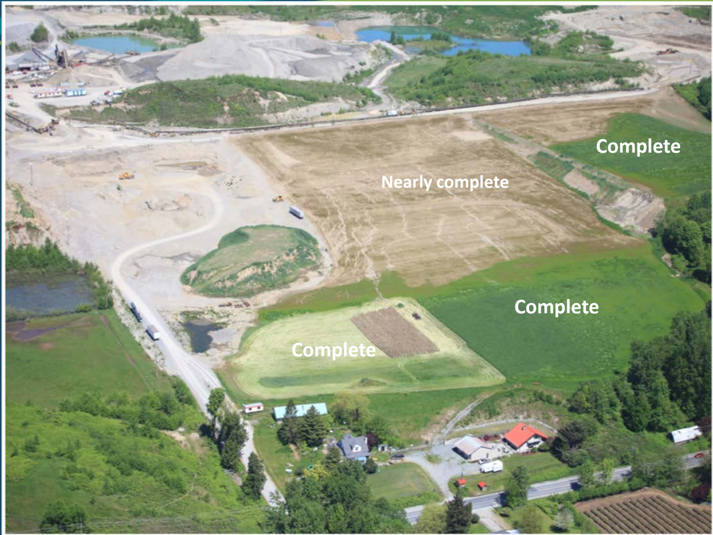
Reclamation in progress, 2012
