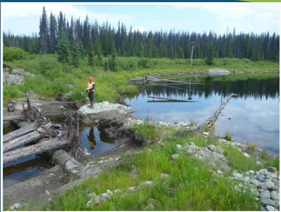
Lower Rainbow Pond constructed in 2013. Note inverted snags and overhanging logs.
