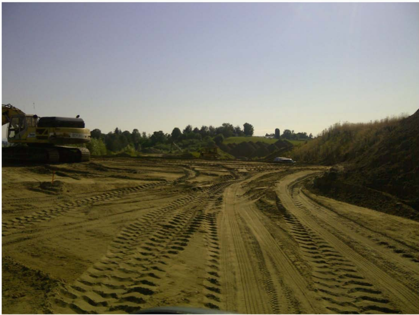
Sand filter layer added across subgrade.
