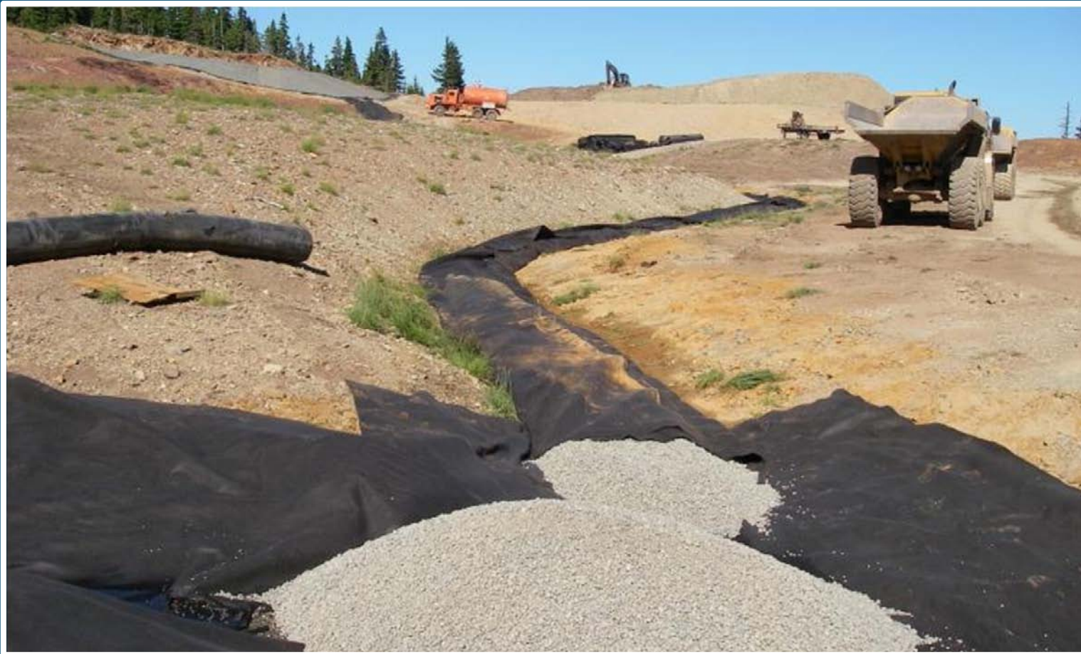
Underdrain Construction
