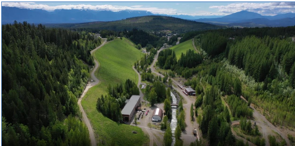
Overview of the Lower Mine Yard at Sullivan Mine
