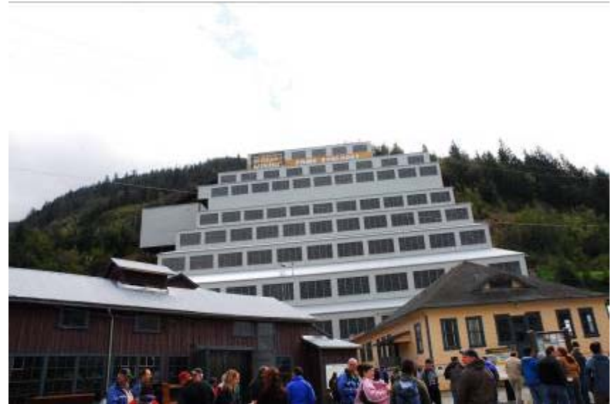
New Britannia concentrator face lift
