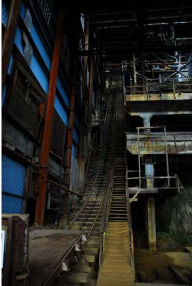
Ore conveyor in concentrator building
