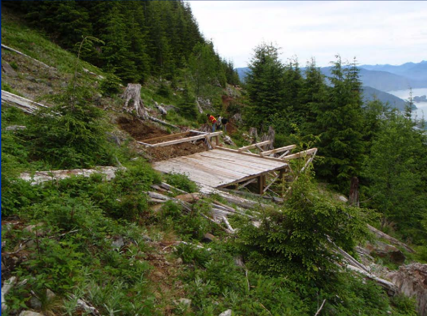
Drill Pad Construction
