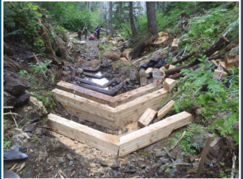
Creek M downstream view of lower fishway prior to remedial works and during construction.
