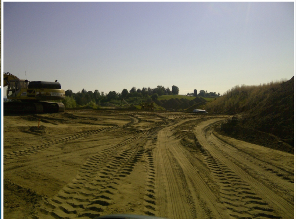
Sand filter layer added across subgrade
