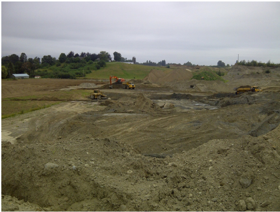
Cut and fill completed to level disturbed area
