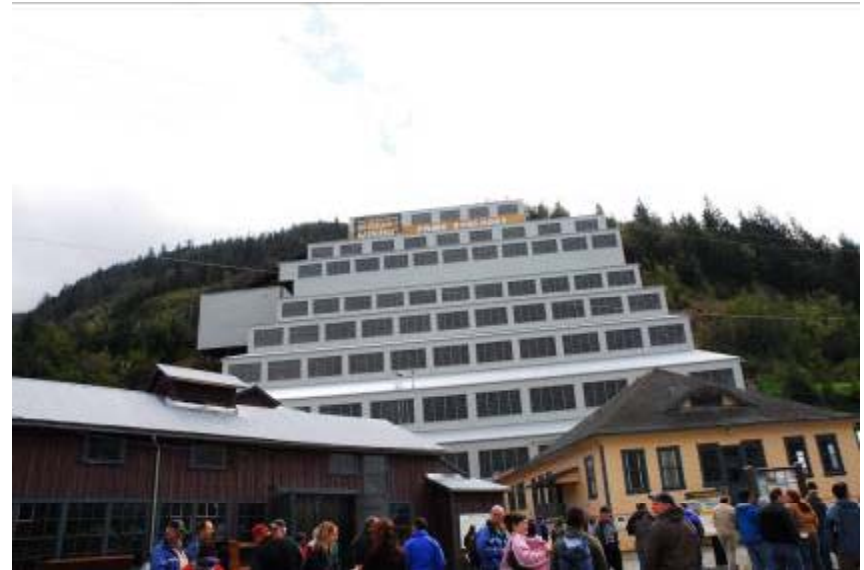
New Britannia concentrator face lift
